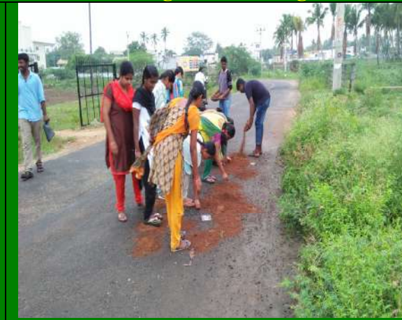
– Road Repairing Work
